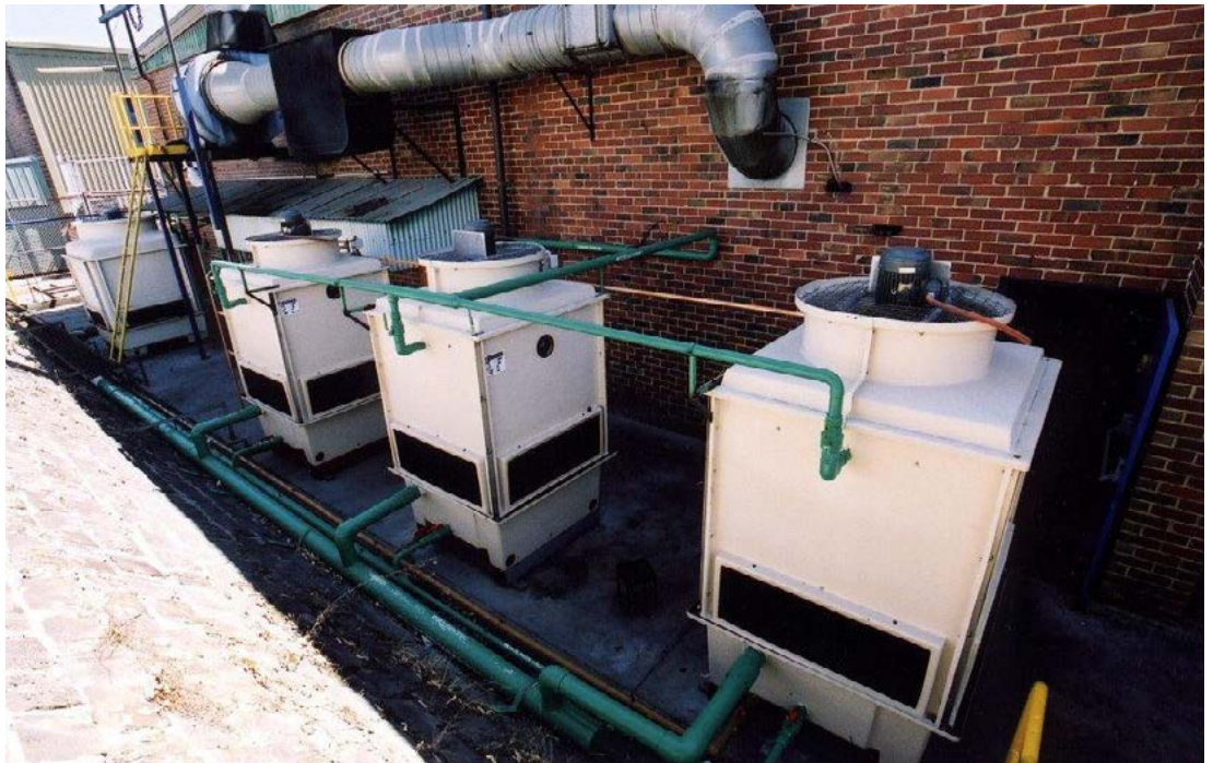
Cooling tower system: A series of inter-connected cooling towers that form part of a cooling tower system.
