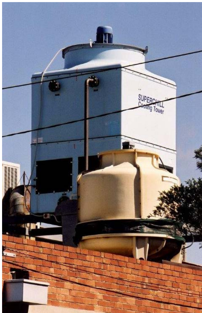
Cooling towers on a rooftop: The tower in the foreground is of fibreglass construction and is often described as a bottle tower. The larger tower at rear is made of metal. Both are induced draught counter flow towers.
