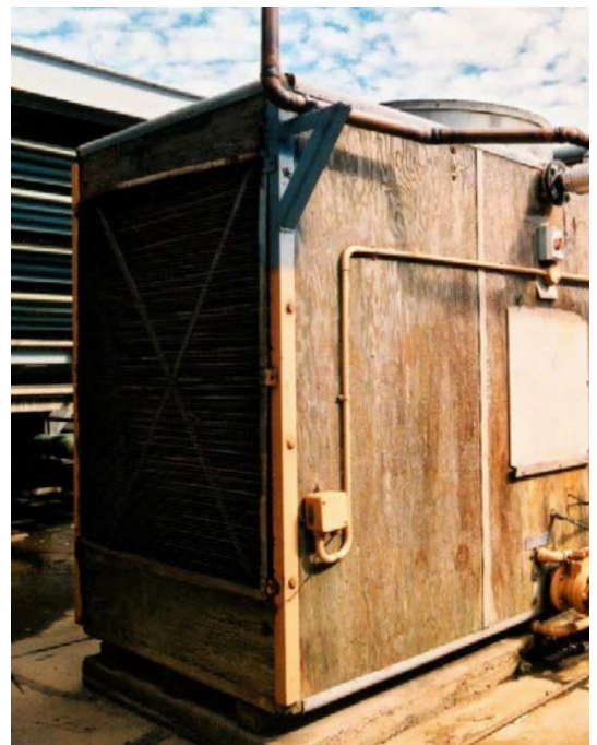
Wooden tower: An aged tower constructed largely of wood
